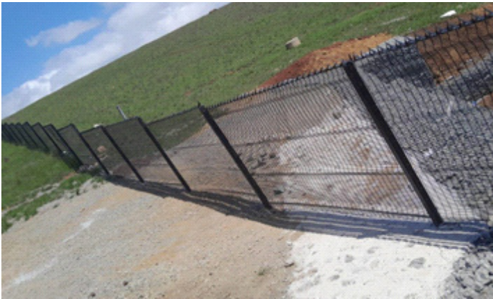
Figure 2. Clear View Fence
