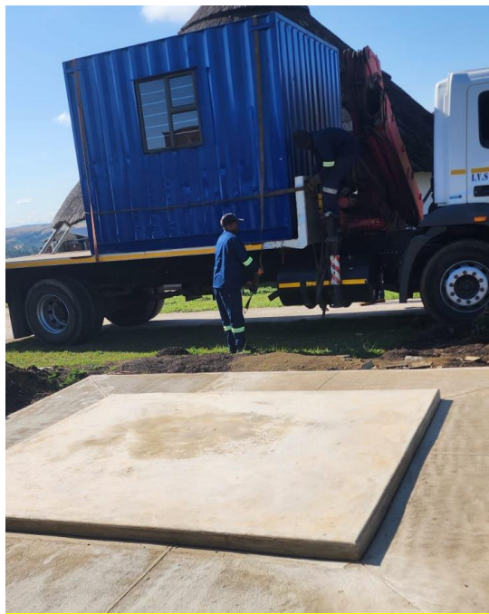
Figure 2. Hazardous Storage Room
