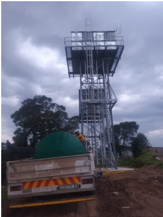
Figure 3. New Elevated Water Tank
