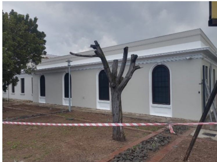
Figure 2. Painting of External Façade
