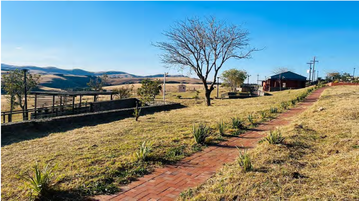
Installation of Paving
