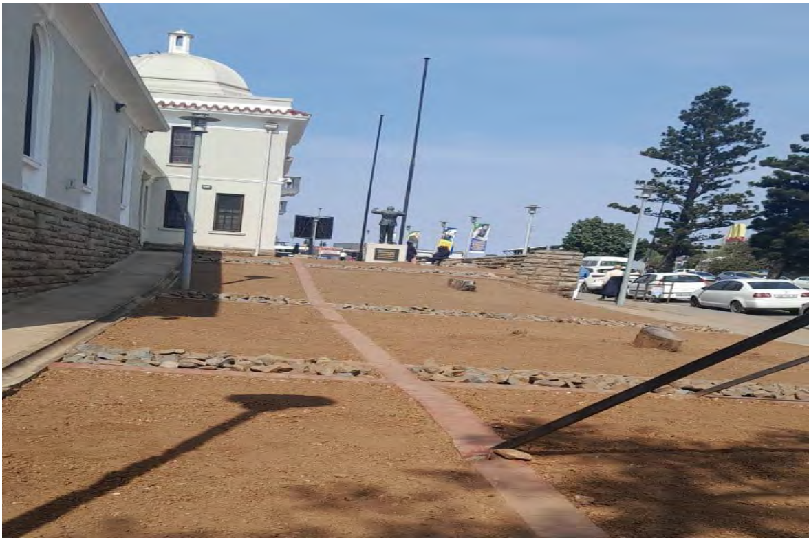
Painting of External Façade
