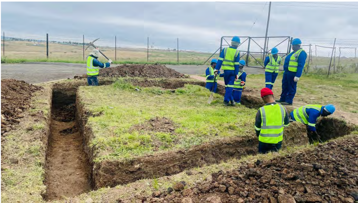
Construction of Guard House
