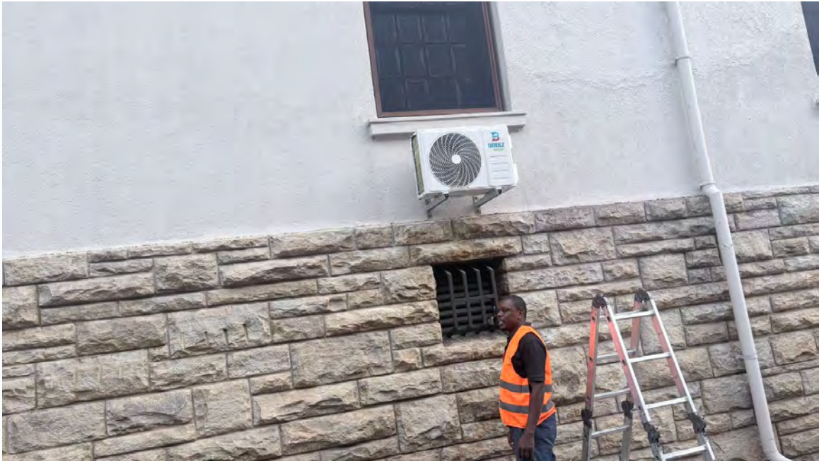
Basement Steel Railings
