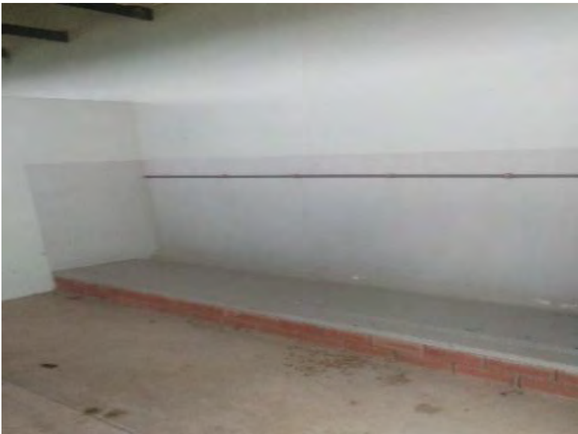
Conversion of Existing Ablution Facilities to Waterborne
