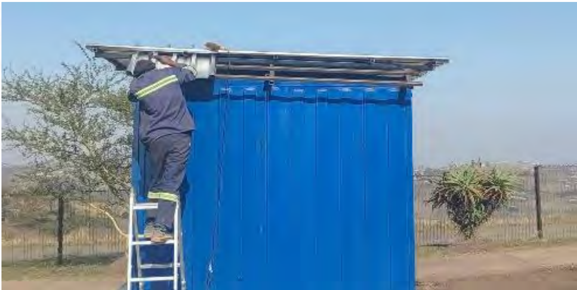
Hazardous Storage Room
