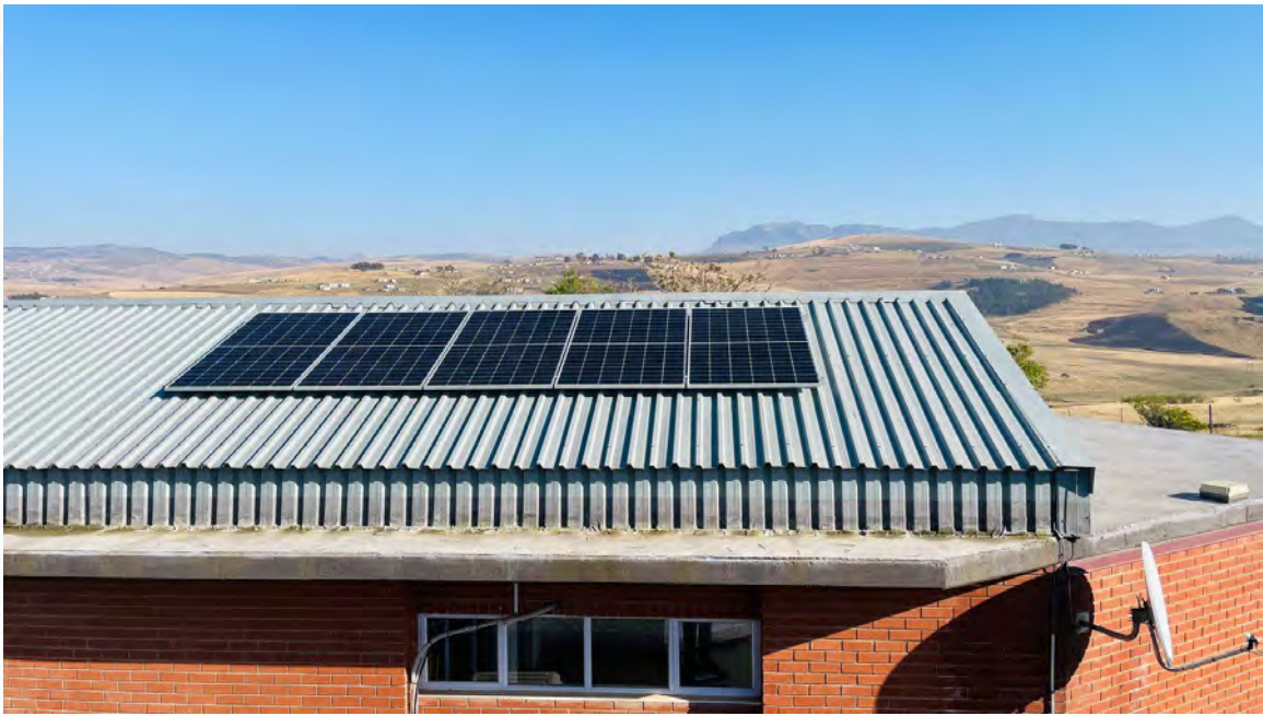
Installation of Solar System
